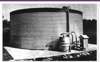
These Open top Water tanks are supplied in kit form ready for installation on site.
